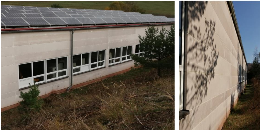
FIGURE 33: VIEW TO THE FACADE OF B.02
