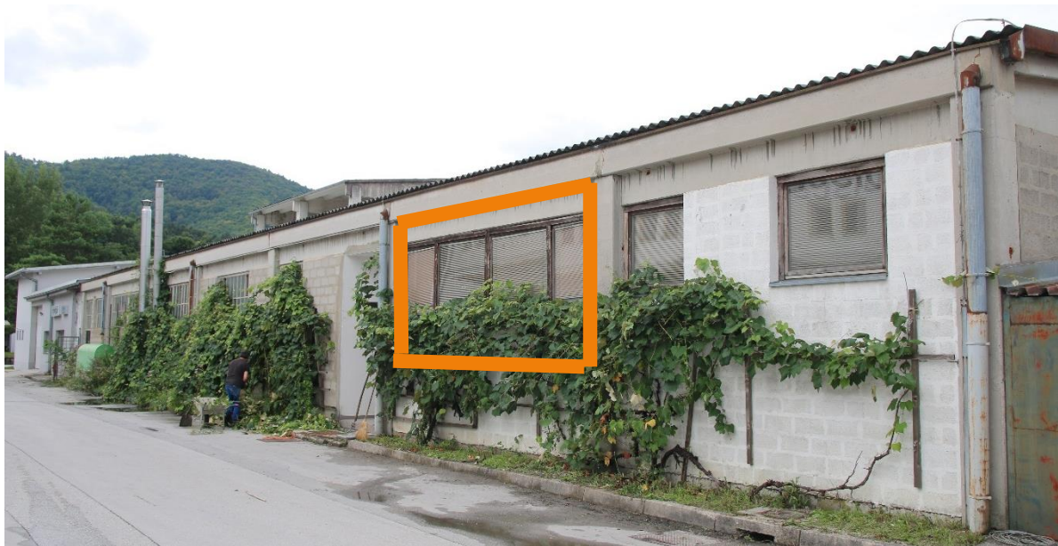
FIGURE 23: VIEW TO THE POSSIBLE INSTALLATION FAÇADE
