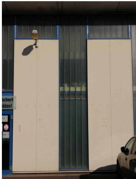
FIGURE 32: VIEW TO THE FACADE OF B.01
